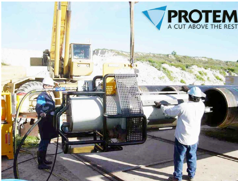
Figure 8 - Application example: Producing a bevel at the end of a pipe, on-site, for an onshore pipeline
